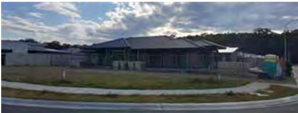
Detached housing construction at North Sandy Beach
